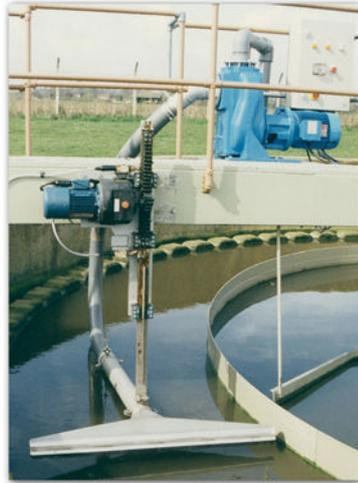
This is employed on radial tanks and is mounted on the rotating half-bridge.
